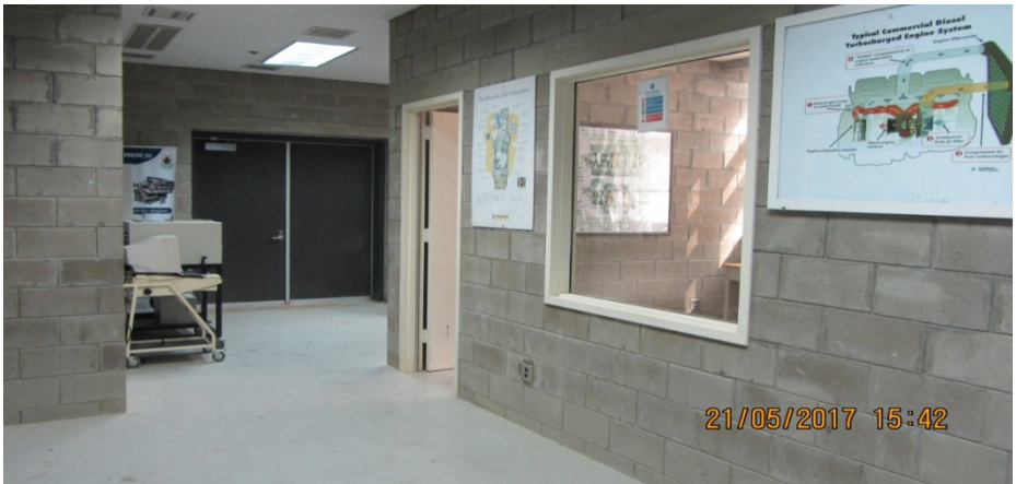
Figure 13.2 General view of the combustion lab Sec-1(right-side)
