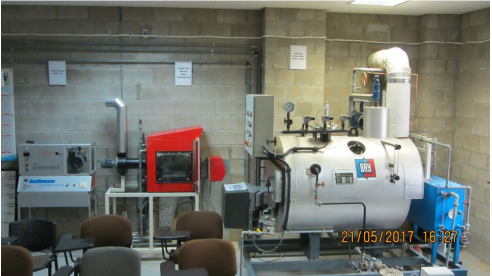
Figure 13.9 Three stopped running equipment need maintenance & resetting: liquid fuel industrial steam boiler (right side), small water heating unit (middle), and burner flame study-unit (left side).
