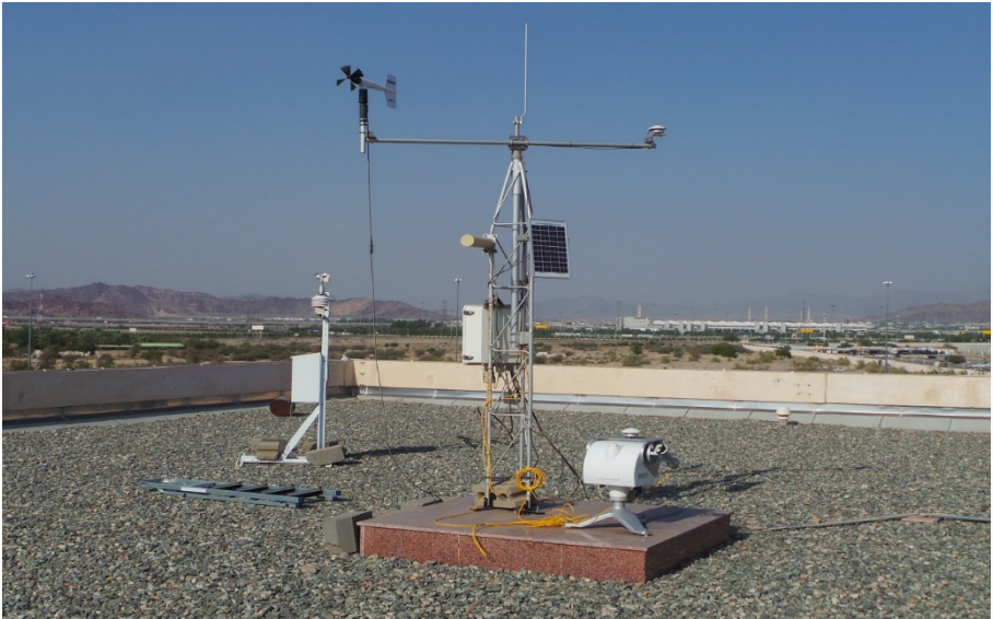
Figure 14.4 Meteorological station, installed on the roof of the solar energy main monitoring room.
