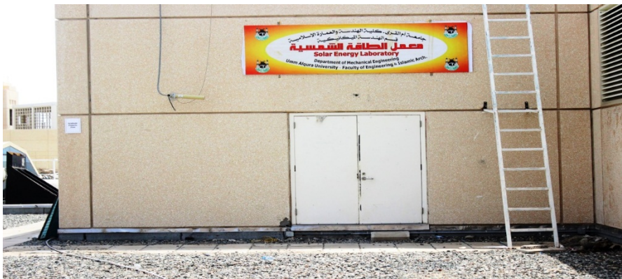
Figure 14.2 General outside view of the solar energy laboratory in 2017
