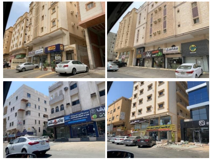
Figure 4. Unmatching colors of shop frame in Almarwah and Alrawdah districts in Jeddah (Author, 2020).
