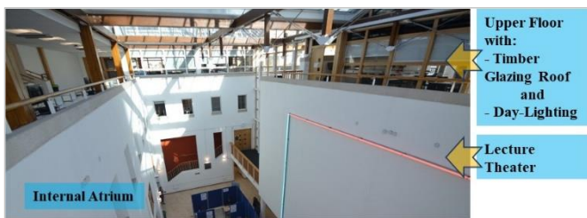
Figure 7 Portland Building Internal Atrium and Upper Floor Details Source Developed by the Authors
