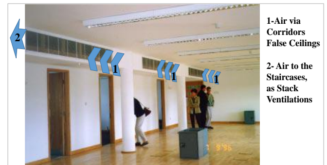
Figure 11 Portland Building Internal Stack Ventilation System
