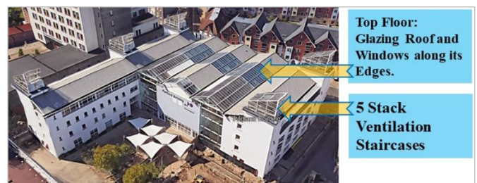
Figure 3 Portland Building External Roof Details
