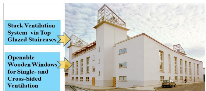
Figure 4 Portland Building External Stack Ventilation Details
