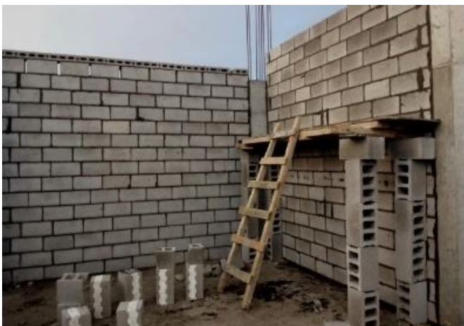
Figure5. Wall system in process for roofing, by researcher
