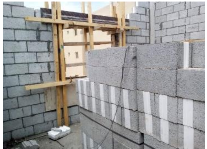
Figure7. Frame wood for beams above the windows, by researcher
