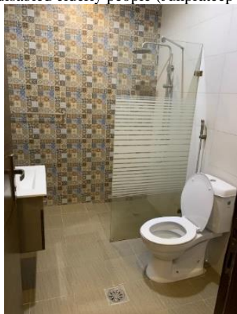
Figure 7: Narrow circulation in toilet with stand-in shower. Source: Author, 2019.
