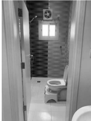
Figure 3: Inner casement door opening. Source: Author, 2019.
