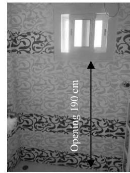
Figure 4: Window opening height in toilet. Source: Author, 2019. Source: Author, 2019.
