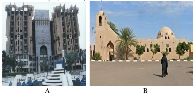
Figure 1: Two Buildings Representing the Main Streams of Contemporary Architecture in the Arab Region - A: Iraq ministry of industry and minerals , B: New Gournah Mosque , Egypt.
