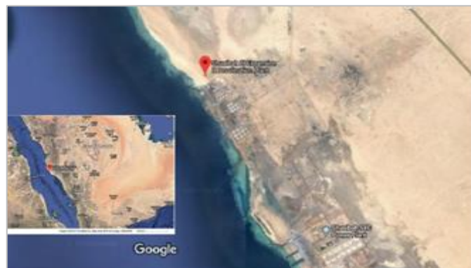
Figure 1. Location of Shuaibah Phase III Power and Desalination Plant in Saudi Arabia.
