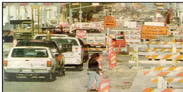
Figure 1: Traditional Open cut excavation: Disturbance for pedestrian, traffic, and environment [8]
