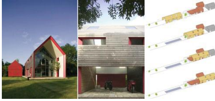
شكل ١٧: Sliding movements of the Sliding House envelope
