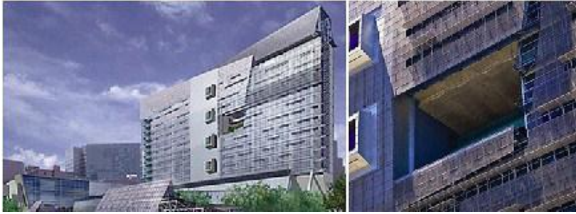
شكل ٢٣: The kinetic double-skins envelope of the San Francisco Federal Building
